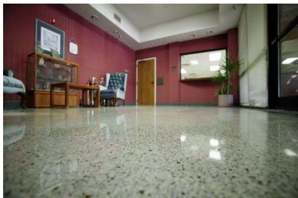
The high shine on Plano's wax-free recycled terrazzo lobby floor is achieved by buffing alone
