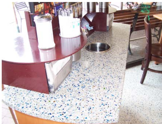
The terrazzo countertops and floors at the Highland Park Village Starbucks feature cobalt blue recycled bottle glass
