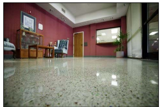
The high shine on this wax-free EnviroGLAS Terrazzo floor is achieved by buffing alone
